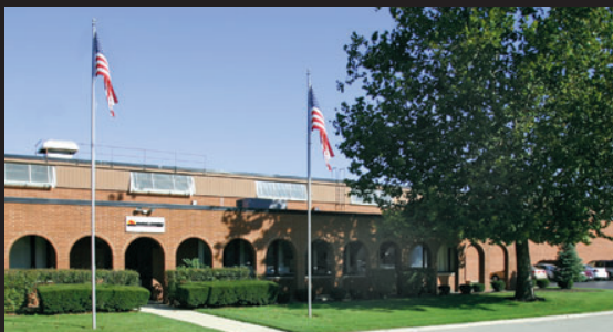
New corporate headquarters and manufacturing facility located in suburban Chicago
